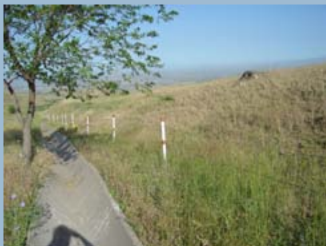
Repaired storm collector
