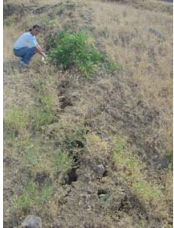
Soil sample taking around the cracks Burial site, 2004
