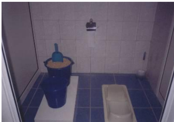
Fig. 9: Ecosan UDD toilet interior. On the left: squatting pan covered with lid and bucket with sawdust. On the right: squatting pan in use (source: AWHEE, 2006)
