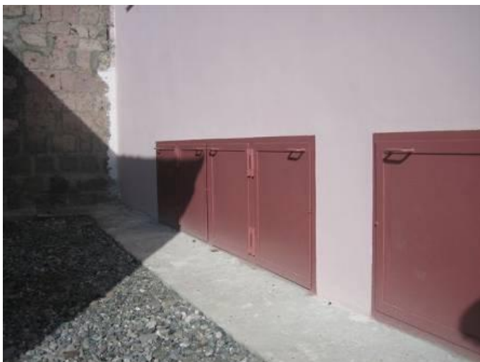
Fig. 12: Faeces collection vaults of UDD toilets (source: WECF, 2006)
