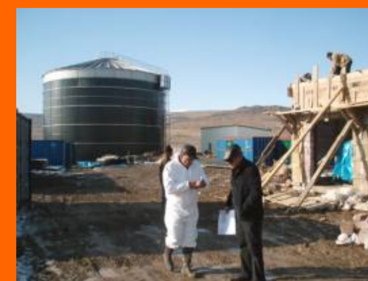
Lusakert Biogas Plant Construction Site
