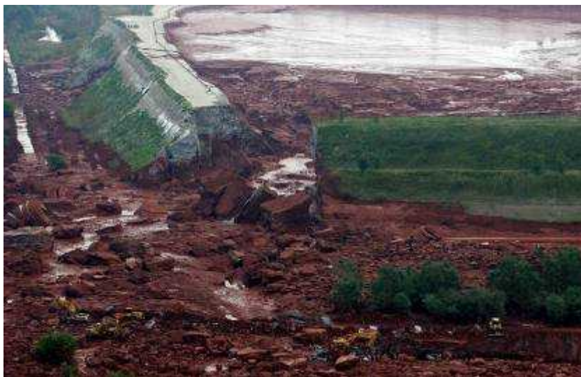
Photo from Hungary that shows the wall that collapsed, releasing the toxic mud. Here you can see the size of the devastation (as compared to trucks at the bottom of the photo)
